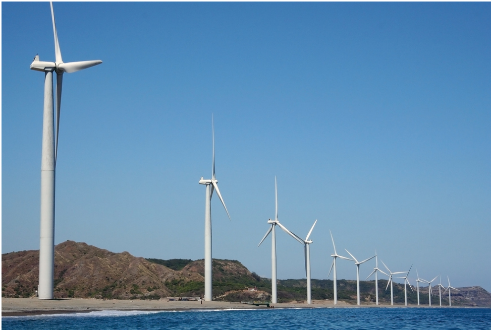
Figure 3.3 : Horizontal Axis Wind Turbines [28]
